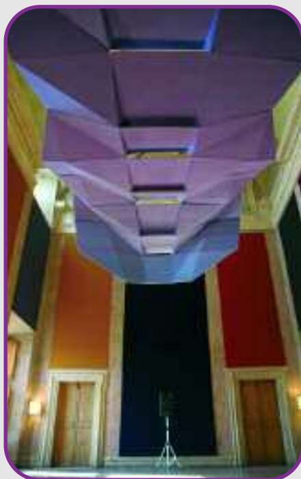
Acoustical domes of variable geometry , Serero Architecture Research Group, Roma, Galleria di Villa Medici
