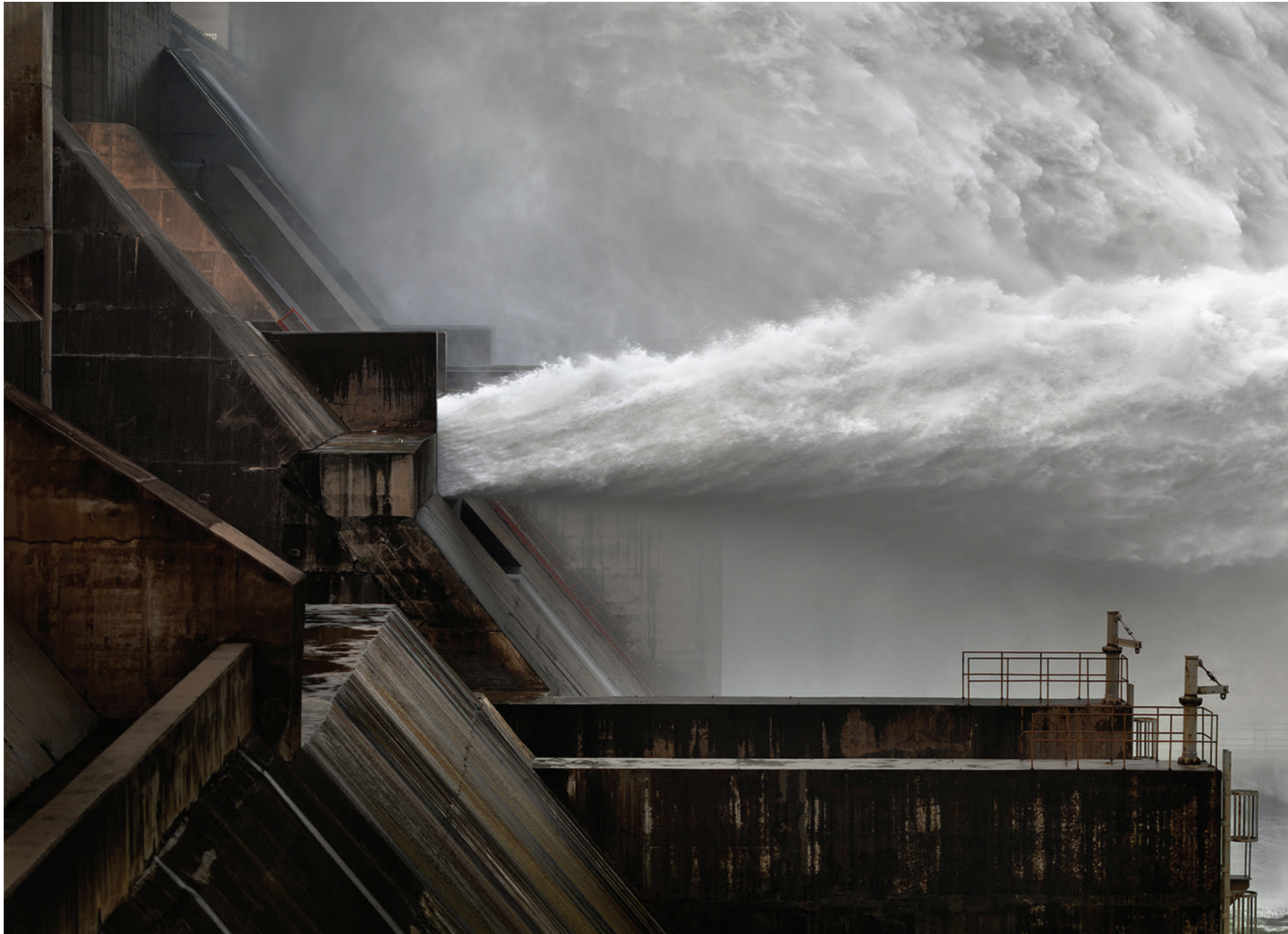
Diga sull fiume Giallo a Henan 2011 © Water by Edward Burtynsky
